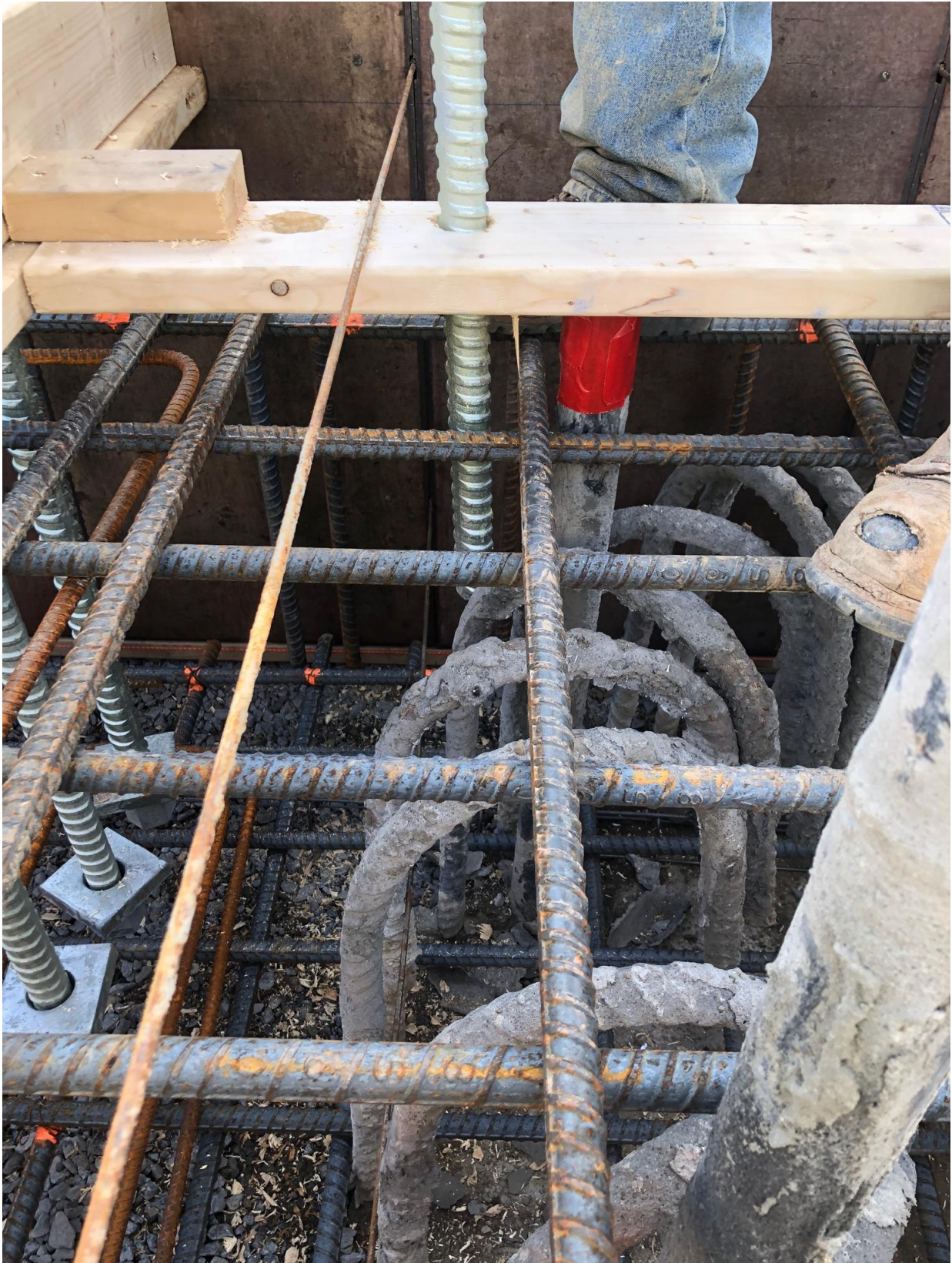
PHOTO #5 – DRILLED SHAFT REBAR CAGE & PRECAST WALL PANEL ANCHORS
