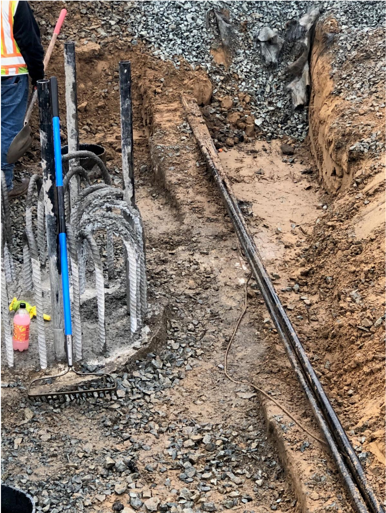
PHOTO #4 – DRILLED SHAFT & STEEL PILE
