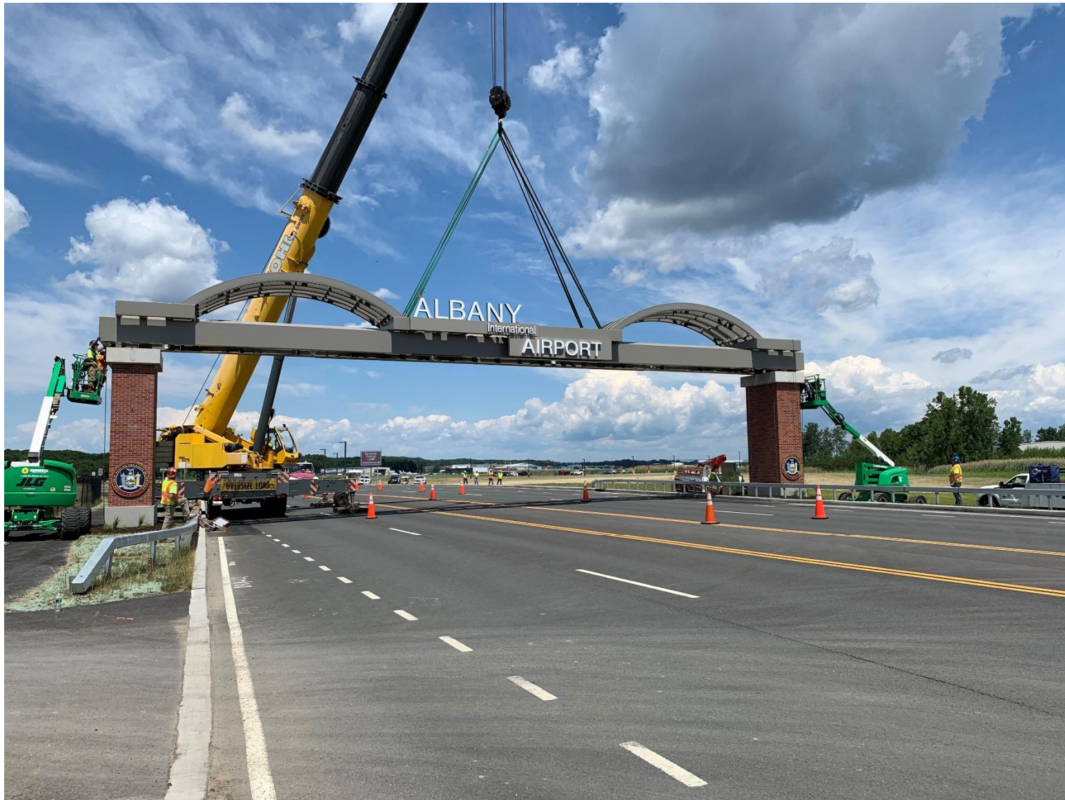
PHOTO #2 – FINAL STRUCTURE – JUNE 26, 2020
